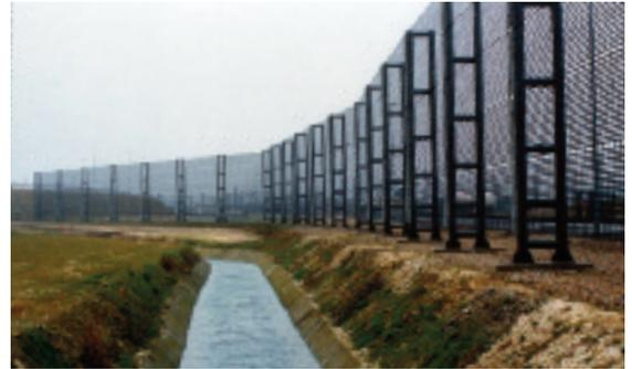
In total 7 kilometres of fence was installed at Coquelles up to a height of 16 metres.
