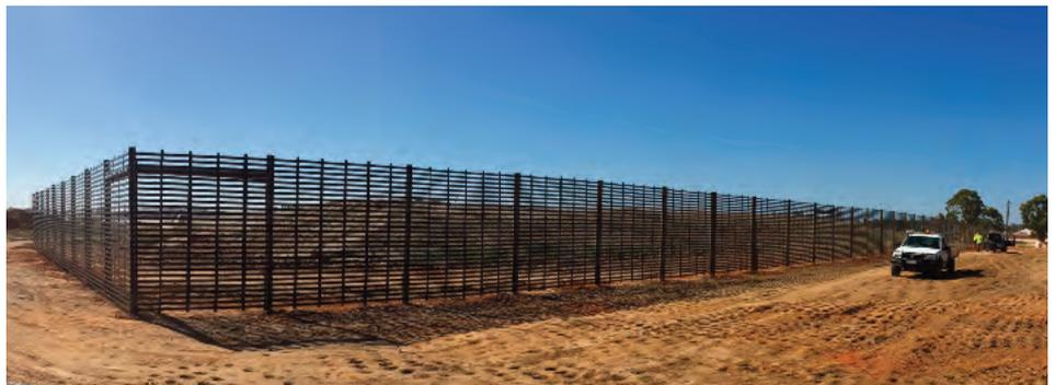
Additionally, they stated "The Parafence™ (with its 45% porosity) is expected to deliver slightly superior spray drift removal than a fence with 50% porosity as specified by the Australian Planning Commission". The Parafence™ system was subsequently approved for use by the City of Swan.
