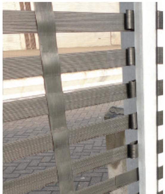
Photograph showing condition of exposed and protected sections of fence (where strips are rolled back - right) after 20 years in service.
