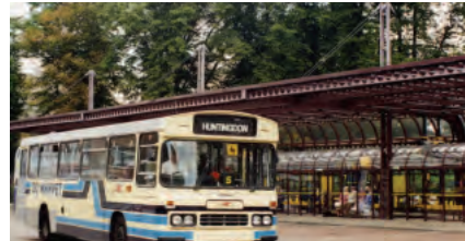
Bus Station roof as viewed following installation in 1991
