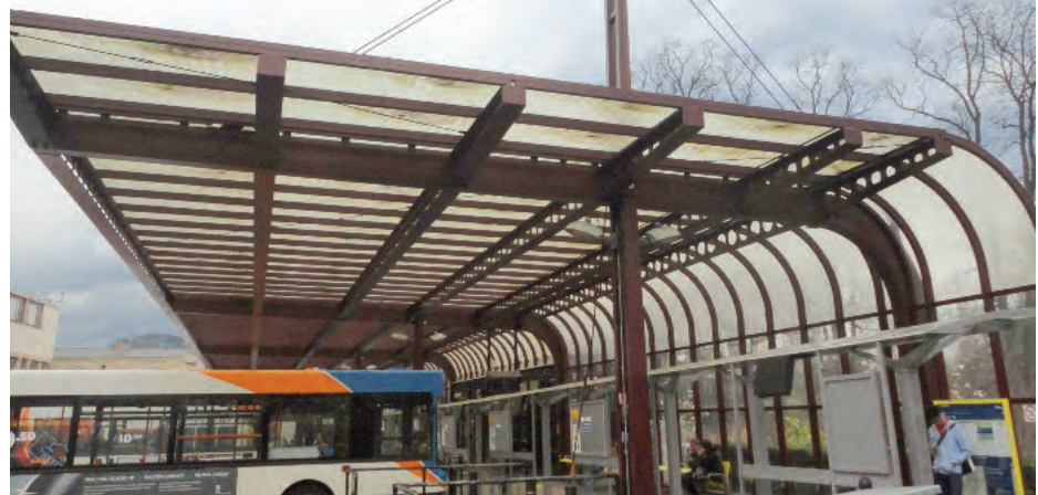
Bus station roof in 2015; 24 years after installation
