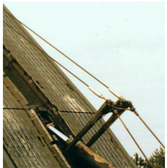
Close up of PARAFIL® launch ties
