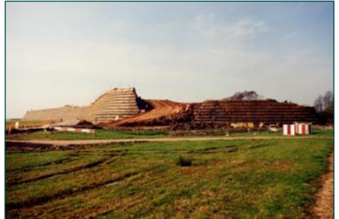
Under construction - from other end
