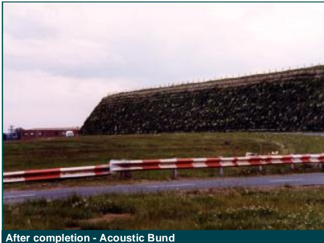
After completion - Acoustic Bund
