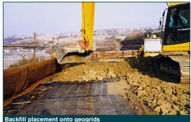
Backfill placement onto geogrids
