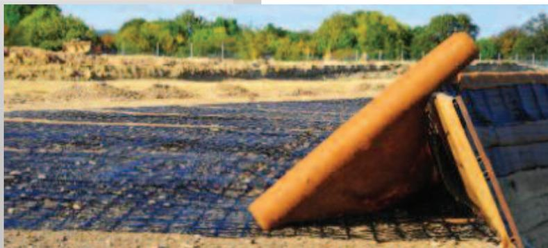
Section showing Biomac C, Paragrid and face formwork
