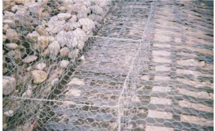
Detail of Paralink® sandwiched beneath Terramesh® unit (unfilled)
