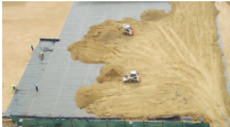
The next layer of compacted decomposed granite was laid on top of the first layer Paralink™
