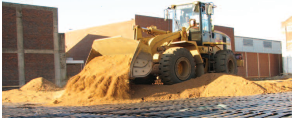
The next layer of compacted decomposed granite was laid on top of the first layer Paralink™
